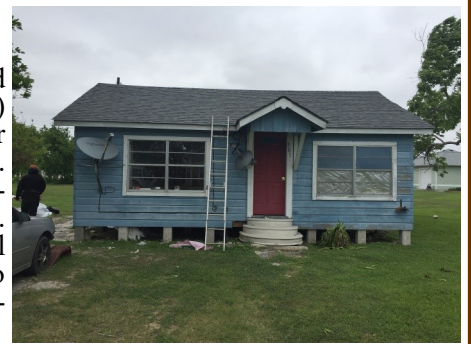
Max's new roof.
