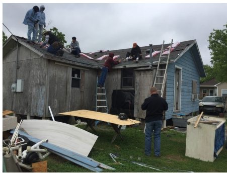
Working on Max's roof.
